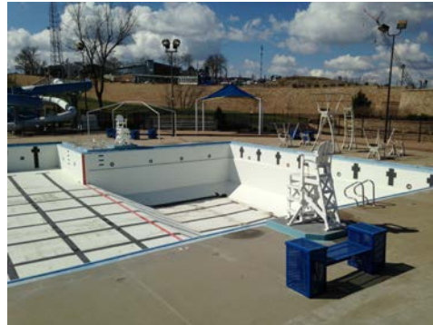
Fig 1. Main Pool Basin
