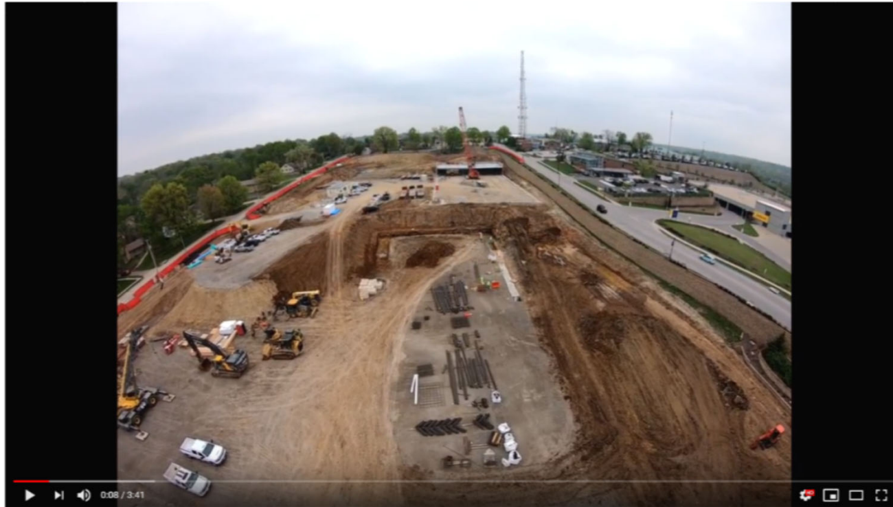
Merriam Community Center Construction: May 2019
