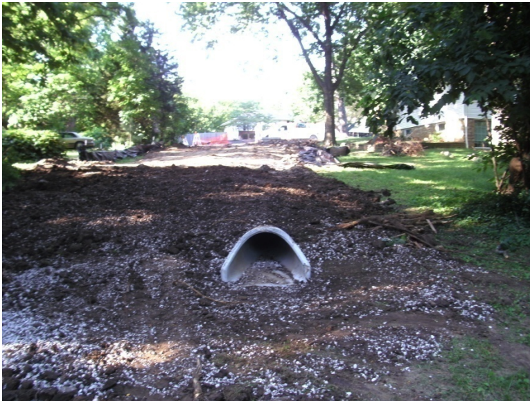
Small storm drain outlet
