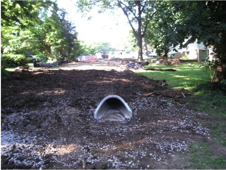
Small storm drain outlet
