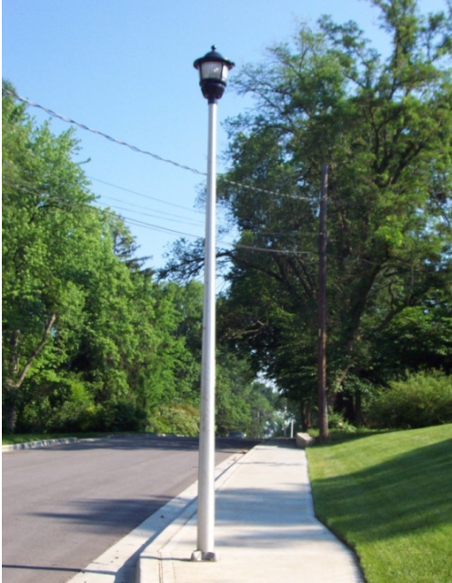
Residential Street light on Goodman north of Johnson Drive
