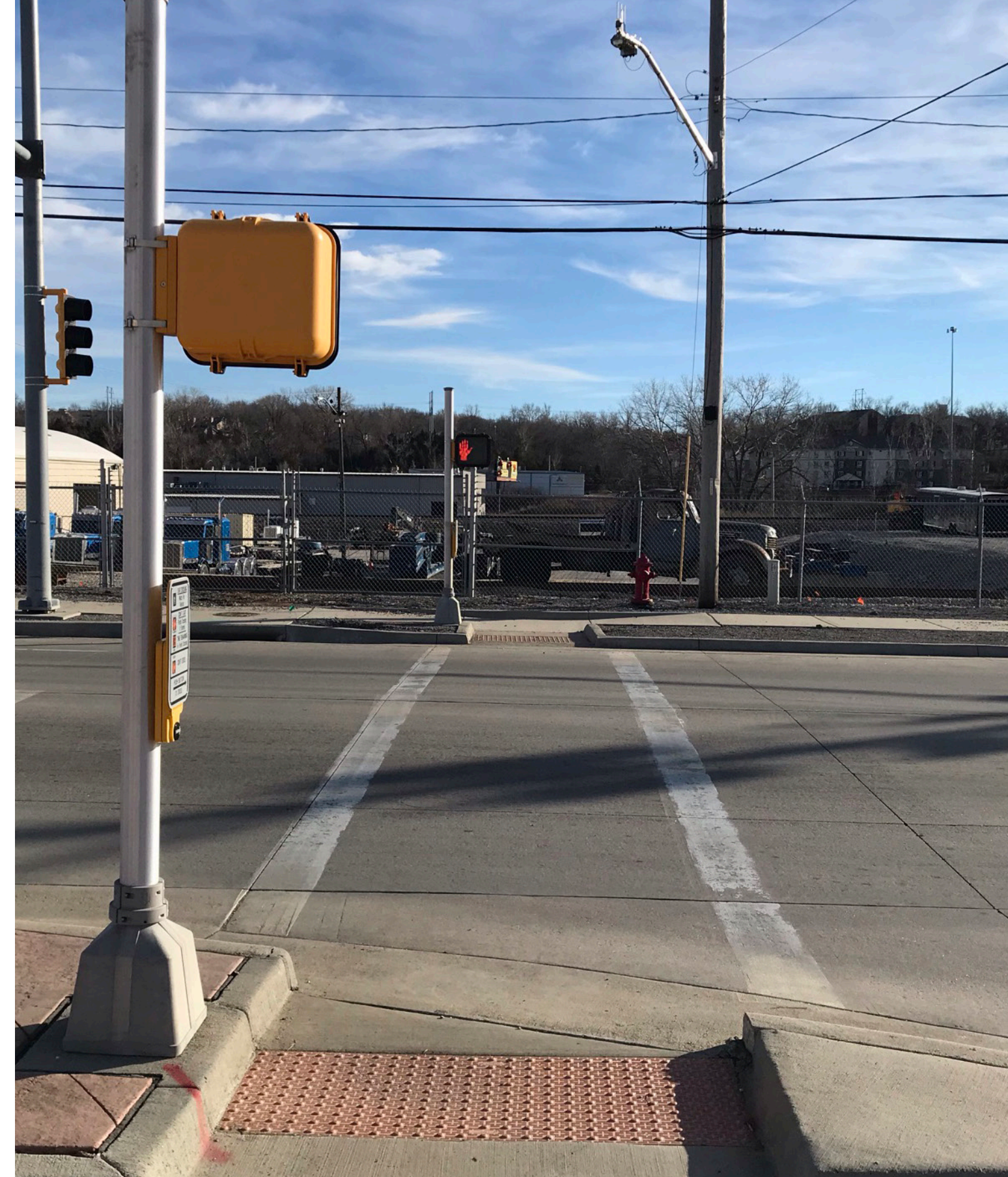
EXISTING CROSSWALK ON MERRIAM LANE IN THE UNIFIED GOVERNMENT
