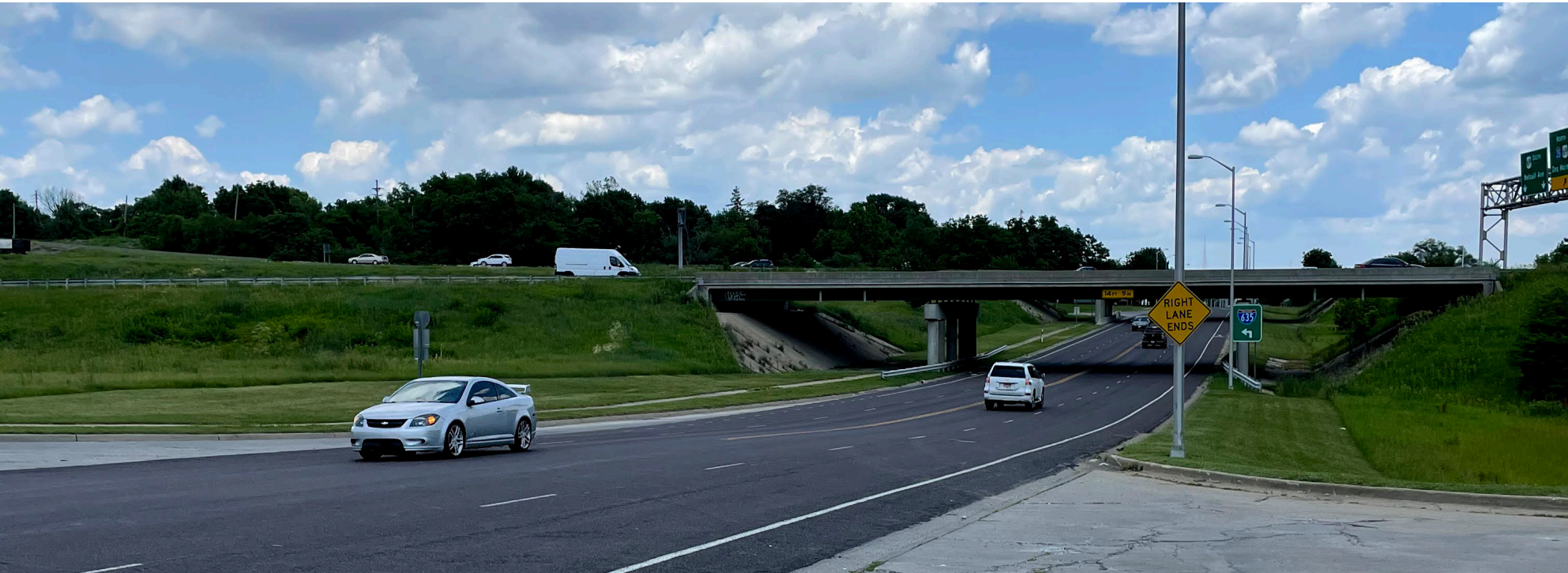
I-635 BRIDGE OVER MERRIAM DRIVE
