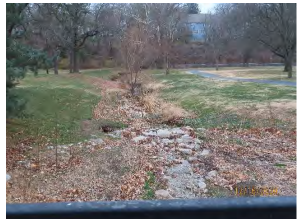
Fig. 6 – There has been a moderate amount of erosion in Quail Creek Park & will be monitored
