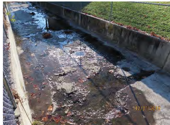
Fig. 4 – Concrete liner is starting to deteriorate and will be monitored.
