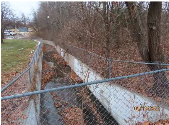
Fig. 5 Brush needs to be removed from fence At 10115 W 47 th St.
