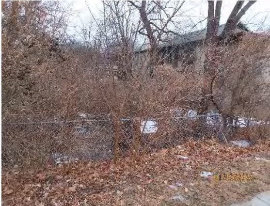
Fig. 1 – Brush needs to be removed from fence. Fence and posts need repair.
