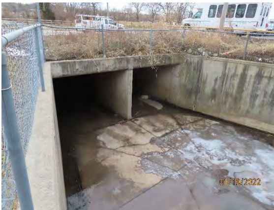
Fig.3 – Sediment has been cleared from under Merriam Dr.
