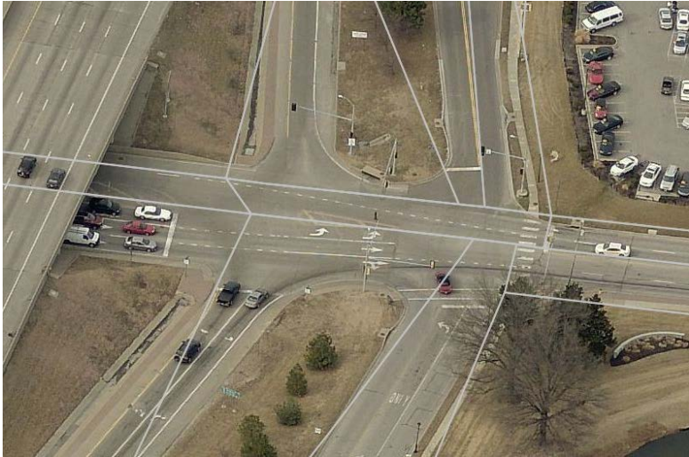
67 th Street & E. Frontage Rd.
