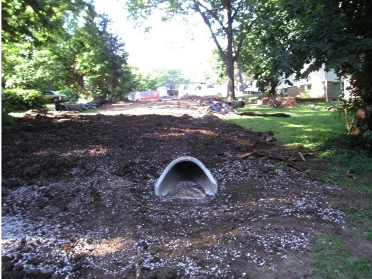
Small storm drain outlet
