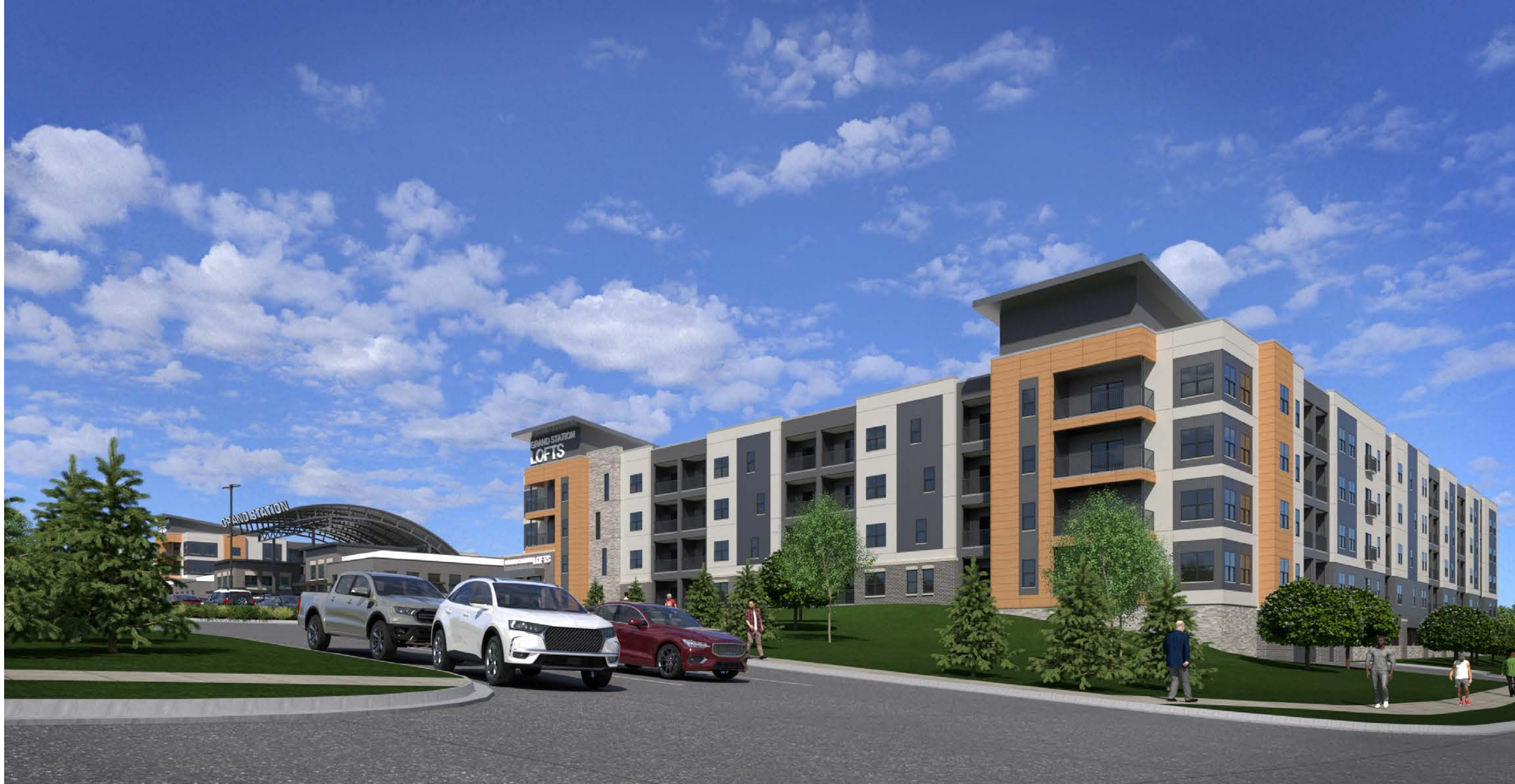
WEST BUILDING – LOOKING SOUTHEAST FROM EBY AVENUE
