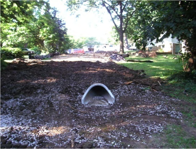
Small storm drain outlet
