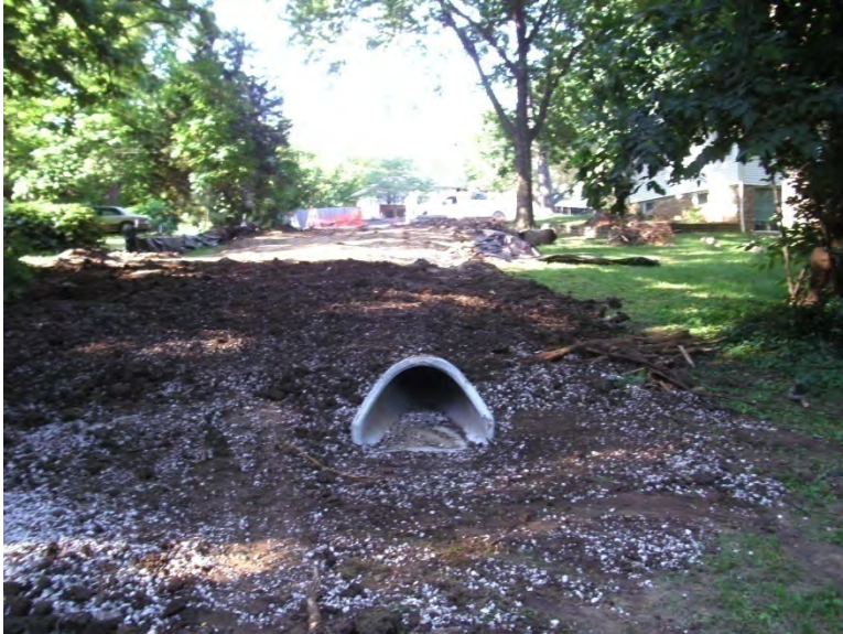
Small storm drain outlet
